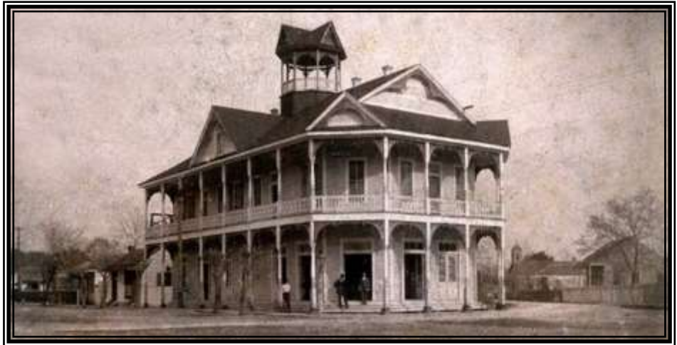
The Gilmore Hotel was located on the corner of Railroad Ave. (Blaize) and Keller St. Bay St. Louis, MS across from the depot.
